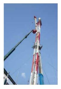
braced framework. The flare burner can be maintained by lowering it by a davit or a crane. The derrick structure allows the installation of several flares together.
